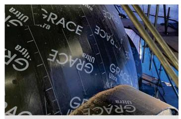
Ice and water shield applied to the dome exterior.
