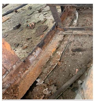
Deteriorated steel at the base of the dome.
