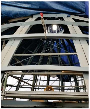
Horizontal bands replacement. Roof sheathing will attach to the horizontal bands.
