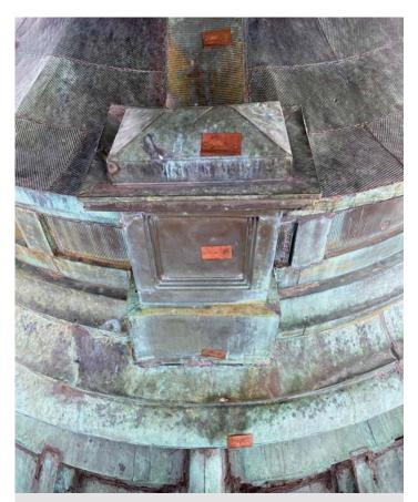
Original copper used as a pattern to replicate the new copper parts. Note the newer copper tags that are affixed to the original copper. A number was assigned to each part and cataloged for reference.
