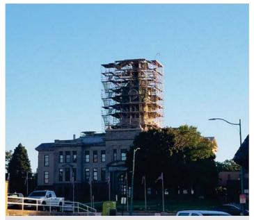
Scaffold installed to complete the dome work. Photo taken prior to it being covered with tarps to allow work through the winter.
