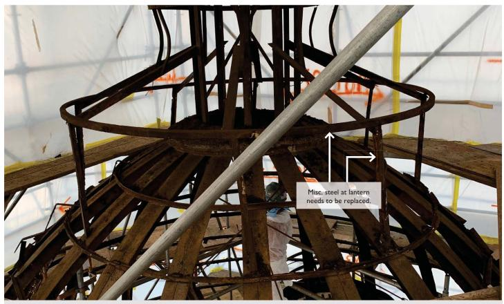
Lantern framing shows corroded steel requiring repair and replacement of sections.
